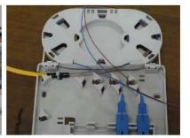
Pic11: install the adaptor and pigtail Pic12: put the pigtail through into the inlet port Pic13: pigtail inserted the
