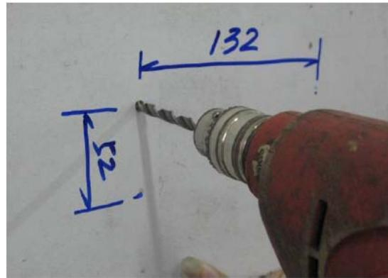
Pic17: the installation hole for the box wall-mount    Pic18: drill the plastic expand hole
