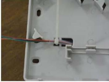
Pic6: dark-routing leads in box fixes by nylon tie
